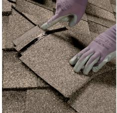
Center over the hip or ridge using the alignment guide
