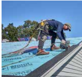
Installs at the eaves and rakes to reduce the risk of shingle blow-off
